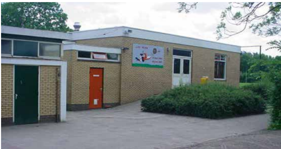
2001 Ingang kantine sportpark Fletiomare West
